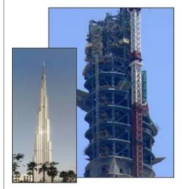
Most of the Burj Khalifa is a reinforced concrete structure, except for the top, which consists of a structural steel spire with a diagonally braced lateral system. 330,000 m3 (431,600 yd3) of high-performance concrete is used throughout the building.
